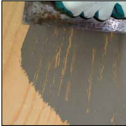
PRO FINE PATCH™ used as a skim coat over plywood
